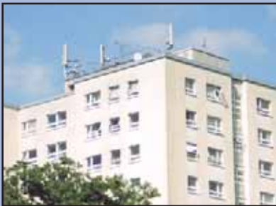
Typical rooftop telecommunications equipment
